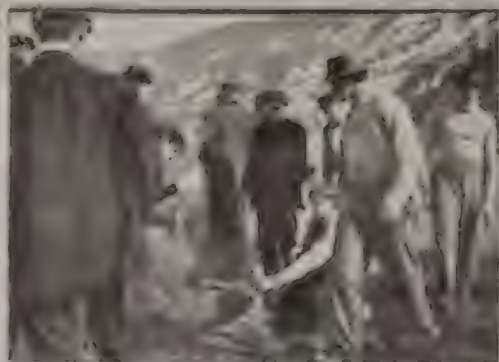
PUTTING IN THE STAKES
